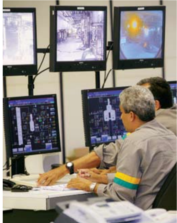
INTEGRATED CONTROL ROOM AT PETROBRAS REFINERY
