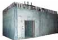
A secure room after filling with concrete mixture and de-panelling
