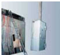
Installation and assembly of Secure door
