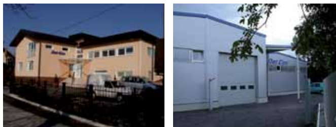
Dat-Con d.o.o. main building and production hall
