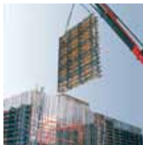
Installation and assembly of wall armouring elements
