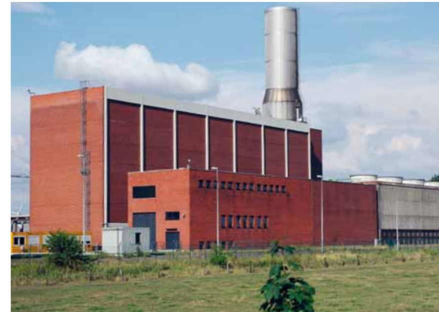
Huntorf Air Storage – Gas Turbine Power Plant
