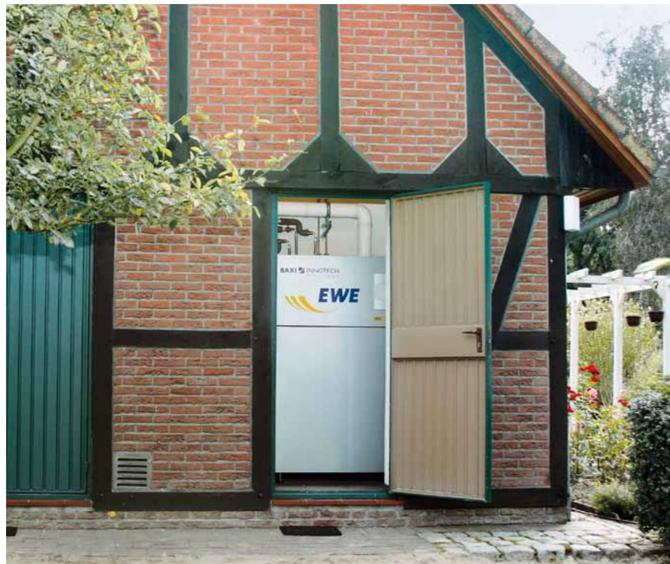
The fuel efficiency of fuel cells employed in combined heat & power mode, exceeds 80%. The electrical power generated by Galileo 1000N unit (a SOFC fuel cell) is 1kW/el, while 2kW/th thermal heat is generated.
