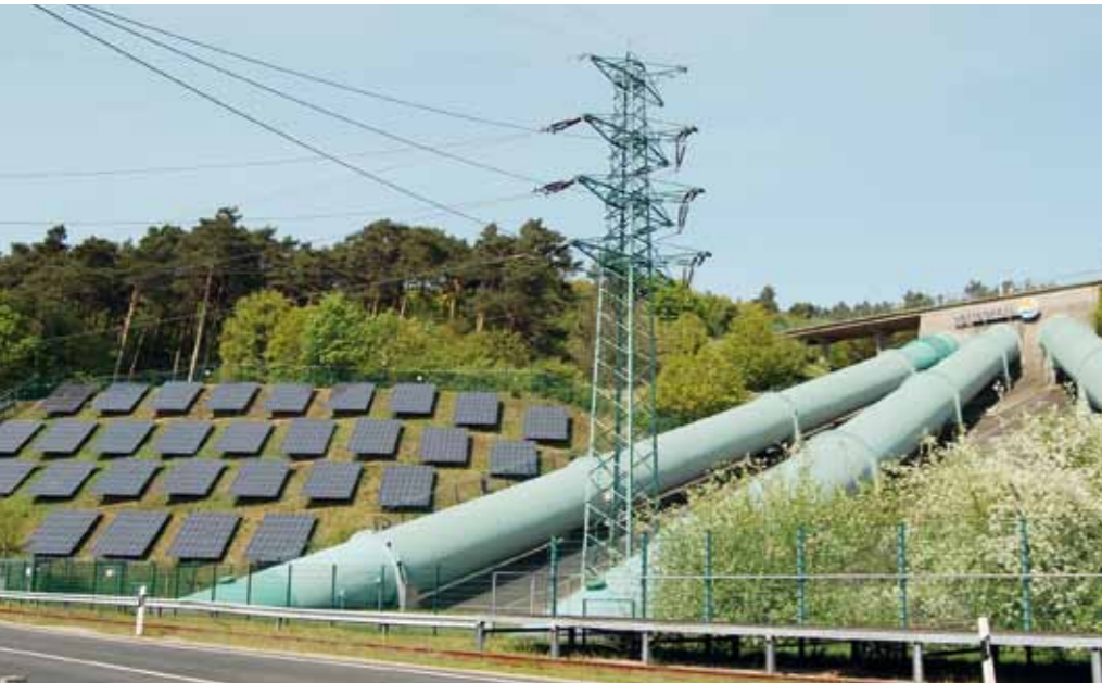
Pumped storage hydro power station in Geestacht, near Hamburg was built in 1958 and is the largest of its kind in Northern Germany. It is part of an environmental energy park with wind and PV-solar power generators. Power rating: 120 MW power and energy storage capacity of 600 MWh. Full discharge capacity reached within 70 seconds. It is activated 4.800 times p.a.
