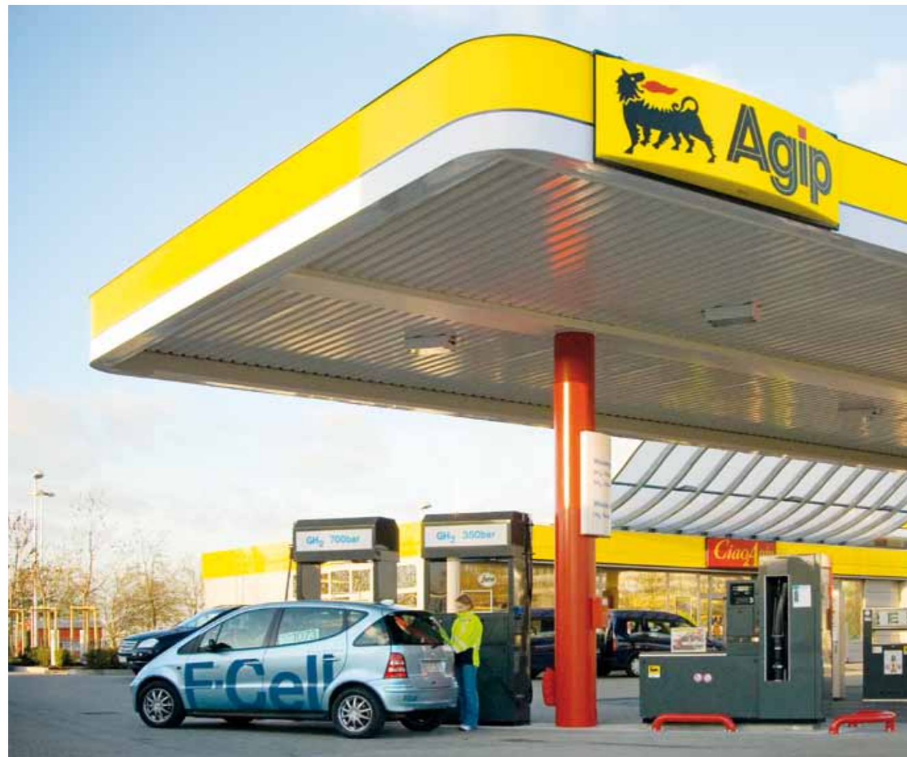
Multi-fuel service station at the Industrial Park Höchst, Frankfurt/Main
