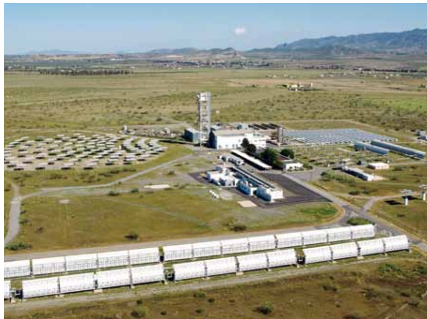
Focal concave mirrors-Heliostat field in Almería The concave mirrors (Heliostats) can be rotated to focus the moving sun onto a central solar receiver at the top of the tower
