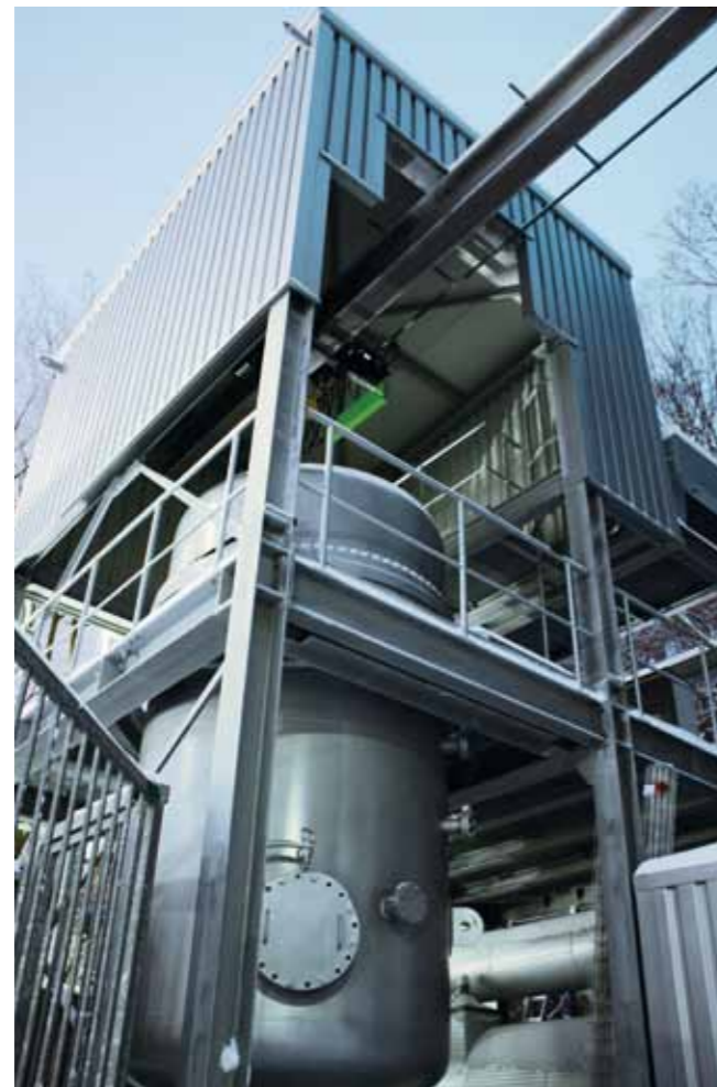
Test facility for the investigation of air-heated regenerator storage designed to cover a large operation range in terms of temperature and pressure, suited to various storage applications, including solar thermal power plants based on air-cooled central receivers, adiabatic compressed air, energy storage (ACAES) or storage-supported combined-cycle power plants in CHP operation.
